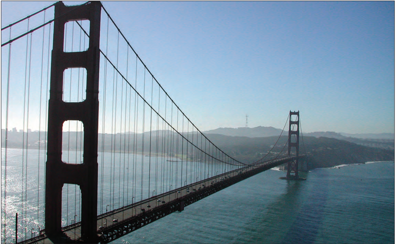
Abb. 1: Golden Gate Bridge in San Francisco, USA
