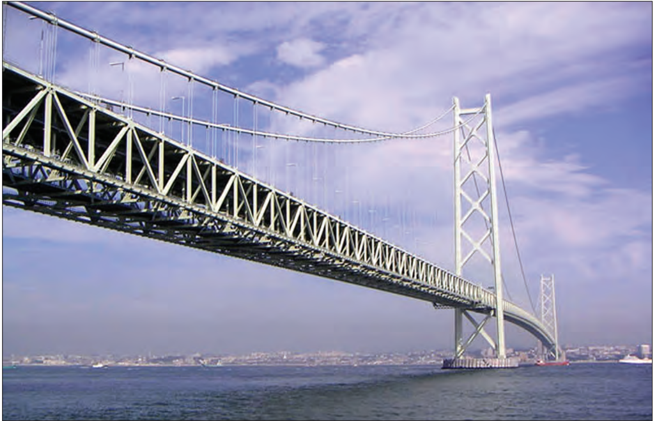
Abb. 1: Akashi-Kaikyo-Brücke, Kobe in Japan
